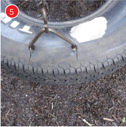
This tire is cracking and should be replaced.
