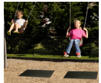
Containment curbs and wear mats help keep loose-fill surfacing materials in place.
